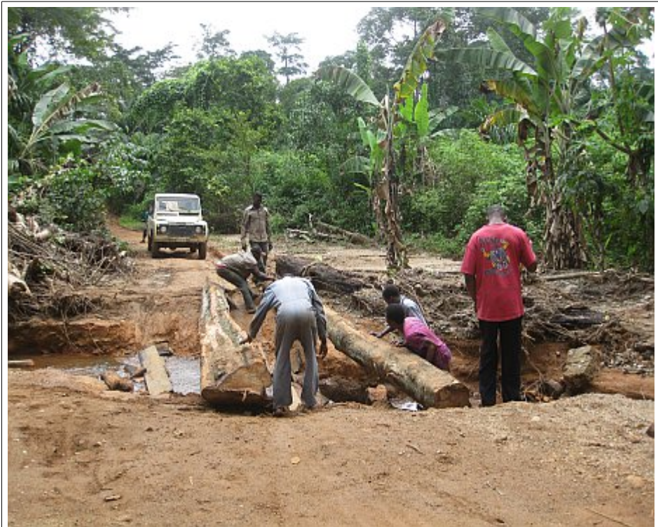
Reconstruction of a bridge organized and paid by Pandrillus
