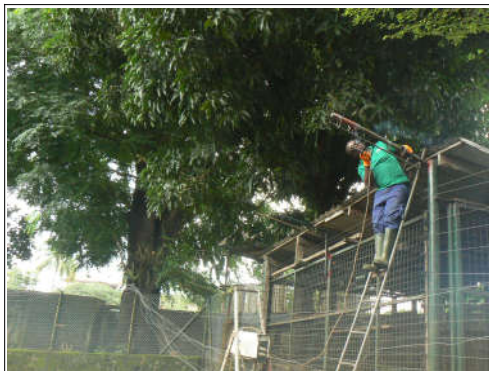
construction of the "overhang" for the drill enclosure at LWC (photo: Peggy Motsch)
